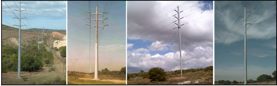
Figure 24: Examples of monopole distribution power line towers.
